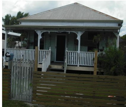
Figure SC6.2.3.8 Illustrates an example of an open front verandah Workers Cottage style
